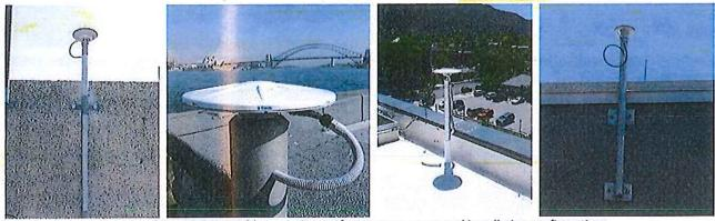
Figure 1. Various examples of Trimble® NetR9® base station roof-top antenna mounted installation configurations.
